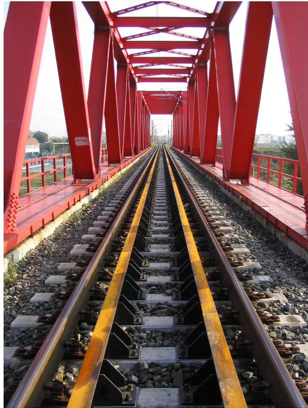
Figure 1.3. An example of a ballasted track form on Arad Bridge in Romania.
