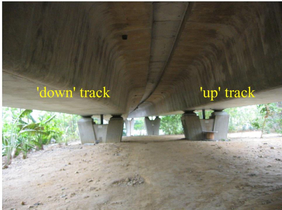
Figure 4.13. The underside of the viaduct consisting of two concrete box sections supporting the deck.
